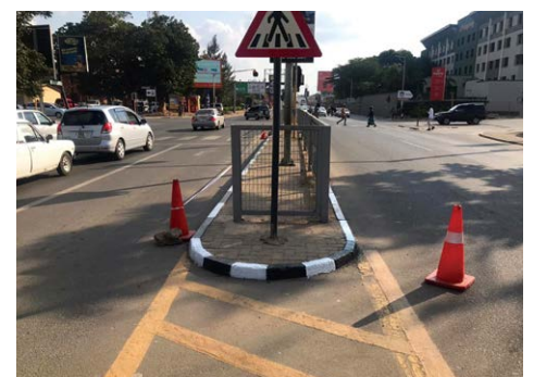
Levy Junction after the work on the safe crossing
